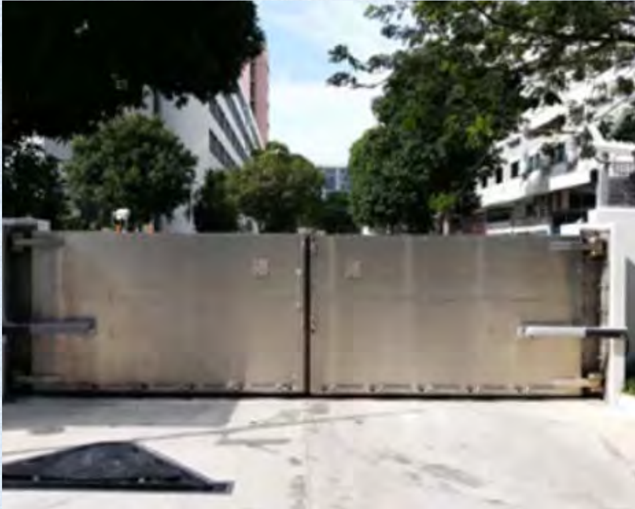
Swing Flood Protection Door
