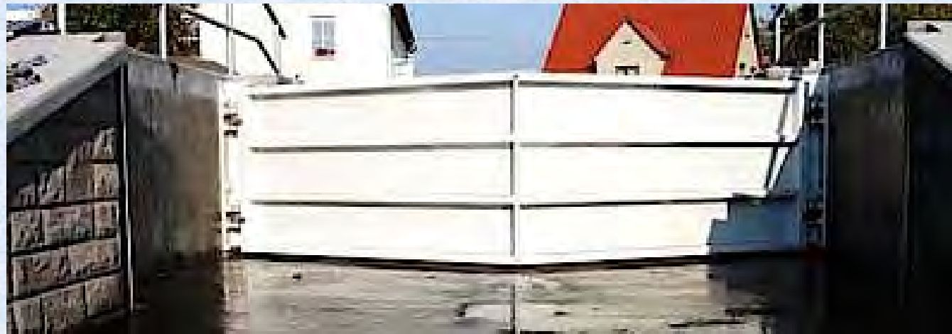
Flood-defence Lock Gate
